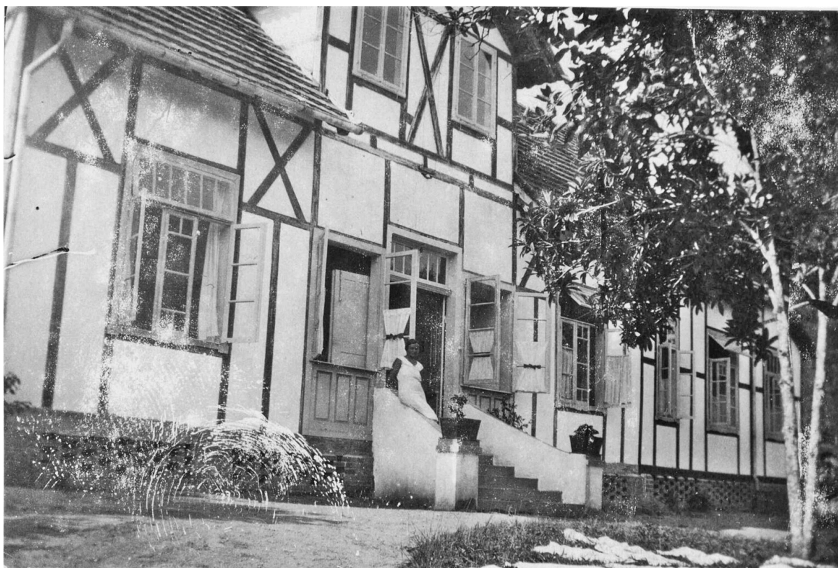
Figura 01: Antigo Hospital Hammonia
